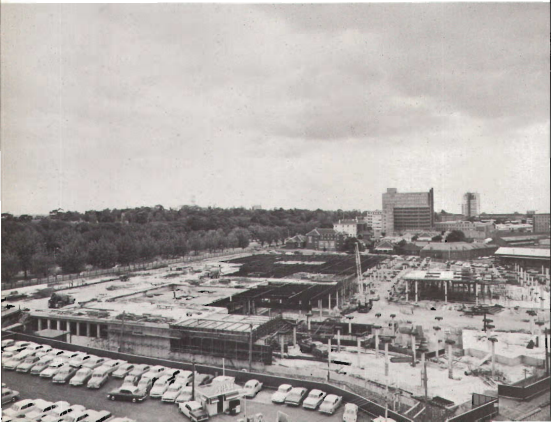
The construction of the car park with its roof as a podium for the new Gallery building.
